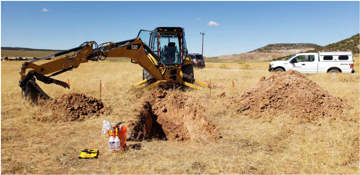
Photo 18. NR-6 test pit excavation showing typical layout with excavated “topsoil” stockpiled on the downhill side of the test pit and excavated spoils on the uphill side. All test pits were backfilled the same day as excavation in 8 in lifts compacted using the bucket of the backhoe.
