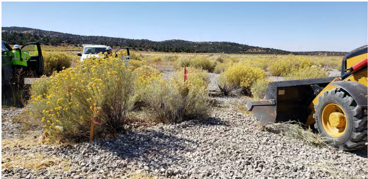
Photo 29. Preparing for excavation of UT-TP2 test pit on the upper tailing impoundment outside of the footprint of the former evaporation cell. This location was the first test pit excavation on the impoundments. Vegetation at UT-TP2 includes rubber rabbitbrush, yellow sweetclover, and Foxtail barley grass.
