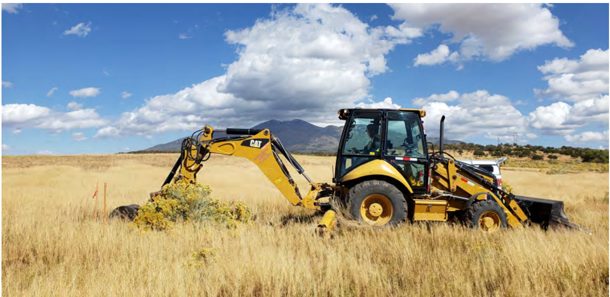
Photo 12. Joseph James (DalMolin Excavating) breaking ground on NR-5 test pit with a rubber-tired backhoe. Vegetation at NR-5 includes Rubber rabbitbrush, sandbur, Tumble and Tansy mustard, and toadflax.
